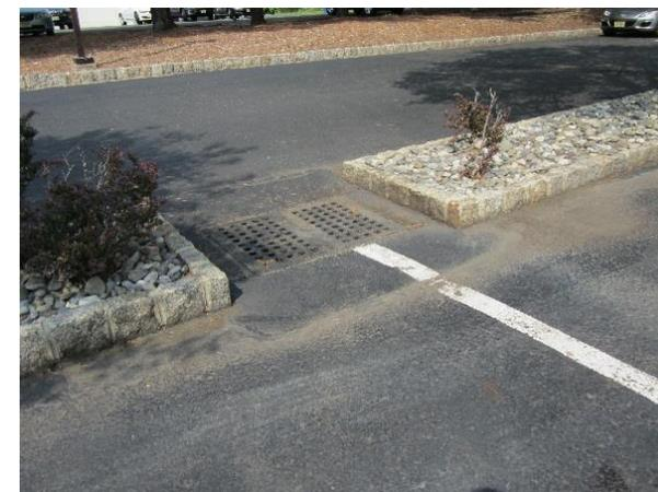
The parking lot is pitched toward the center. Parking spaces in the center of the lot can be repaved with porous asphalt to help manage stormwater. A preliminary soil assessment suggests that more soil testing would be required before determining the soil's suitability for green infrastructure.
