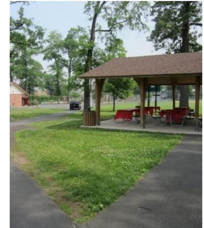
Gutters and downspouts can be installed on the pavilion at the center of the park. A bioretention system can then be installed in the adjacent turf grass to capture, treat, and infiltrate runoff from the roof. A preliminary soil assessment suggests that the soils have suitable drainage characteristics for green infrastructure.
