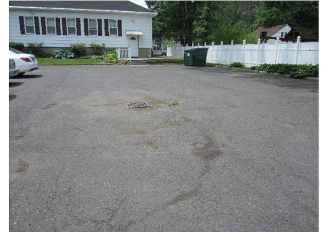
Parking spaces can be replaced with pervious pavement to infiltrate runoff. A rain garden can also capture, treat and infiltrate stormwater. A preliminary soil assessment suggests that more soil testing would be required before determining the soil's suitability for green infrastructure.
