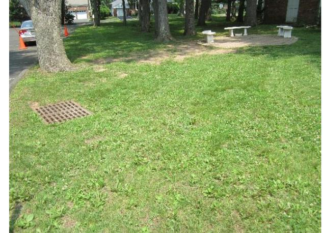
Downspouts on the northeast side of the building are already disconnected into adjacent lawn. On the northwest side, a rain garden could be installed where a catch basin is currently located, in order to capture, treat, and infiltrate roof runoff. A preliminary soil assessment suggests that the soils have suitable drainage characteristics for green infrastructure.
